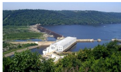
Holtwood hydro plant
